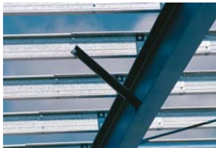
Lap, cleat & fly bracing detail
