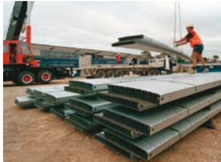
Efficiently bundled and stacked
